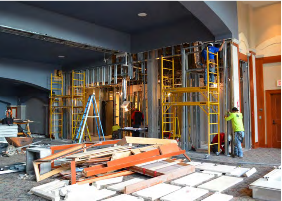
Renovation of the IMAX® Theatre and lobby in progress.
